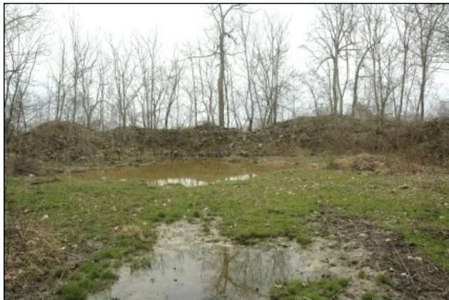
FIGURE 15. AREA WHERE STONES HAVE BEEN REMOVED FROM THE MOUND.
