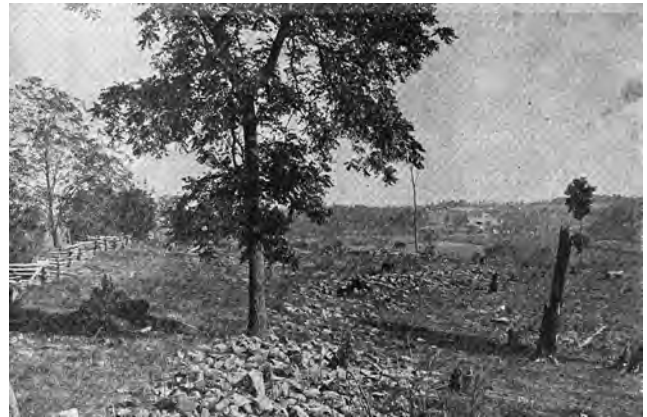
FIGURE 9. 1902 PHOTOGRAPH OF EASTERN WALL. FOWKE
