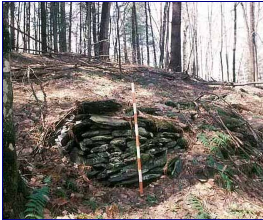
Figure 6: Terrace Fill at Southbridge VT
