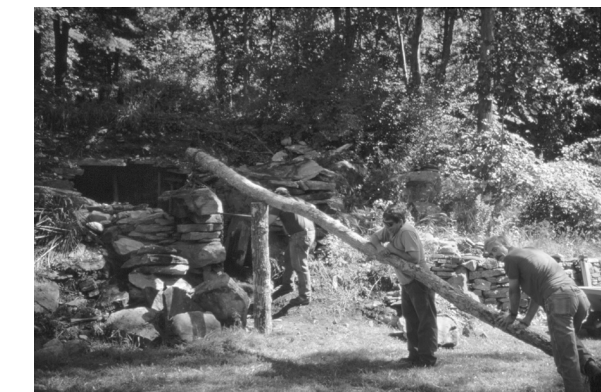
FIGURE 12. 30-FOOT LEVER HOISTS 500 LB. LINTEL.
