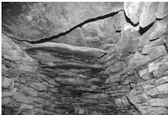
FIGURE 2. CRACKED CAPSTONES.
