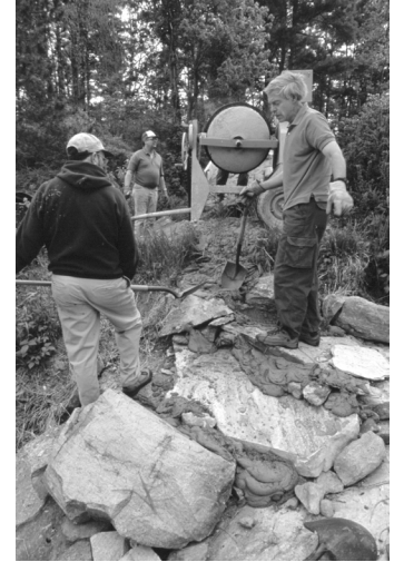
FIGURE 15. CEMENTING GAPS TO PREVENT WATER SEEPAGE.
