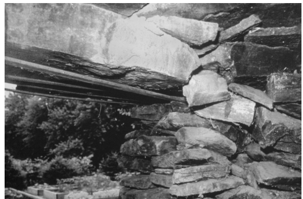
FIGURE 3. IRON RODS SUPPORT BROKEN LINTEL.
