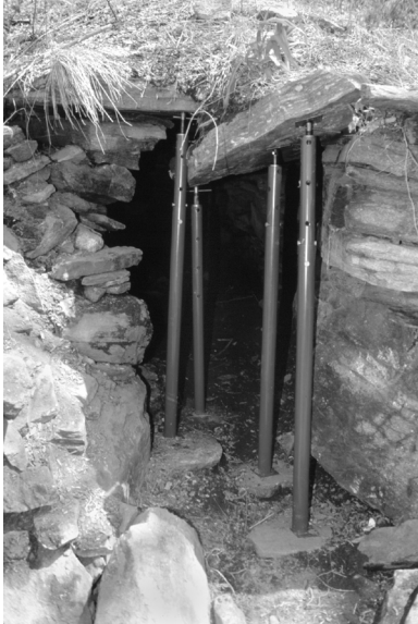
FIGURE 5. TEMPORARY LALLY COLUMNS.
