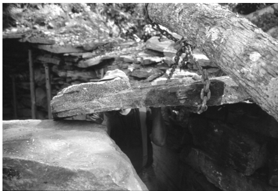
FIGURE 13. MANEUVERING LINTEL INTO PLACE.
